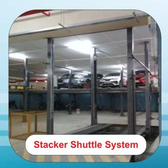
Stacker Shuttle is the optimized design recommended for multiple car parking with multiple entry/exit with peak hour management system.
